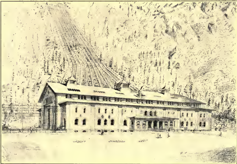
WHITE RIVER POWER PLANT, 60,000 H.P.
